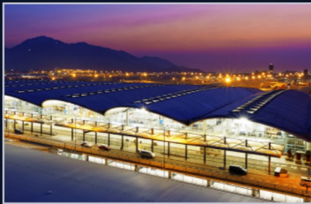
Hong Kong International Airport
